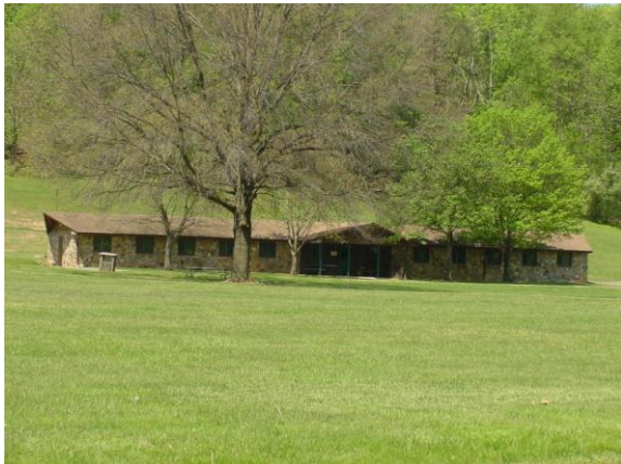
Outside View of Cottage
